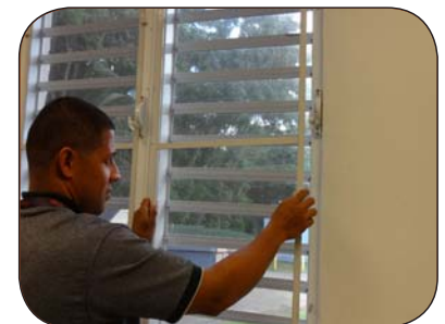
Install or repair window & door screens.
